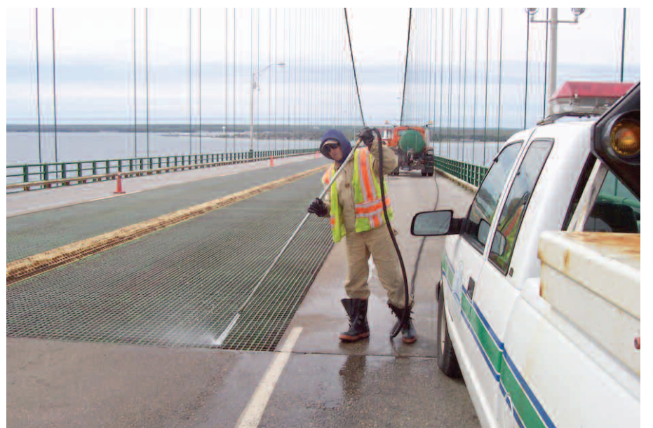
Mackinac Bridge Authority (MBA) employees sweep and wash off sand and road salt that is tracked onto the bridge and accumulates in nooks and crannies each winter. (MBA photo)
